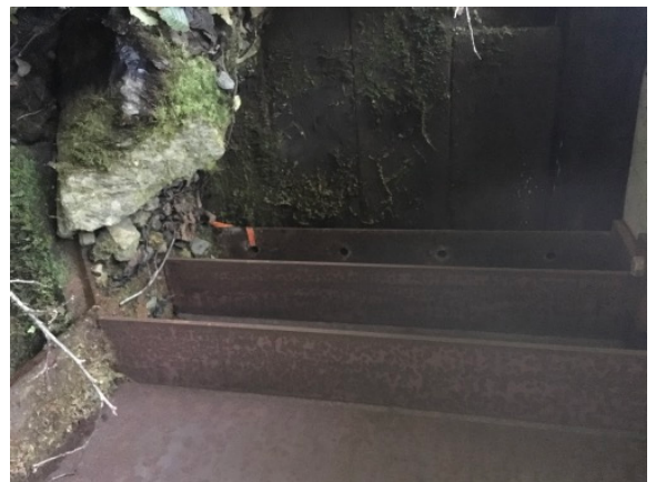
Ballast timber connection
