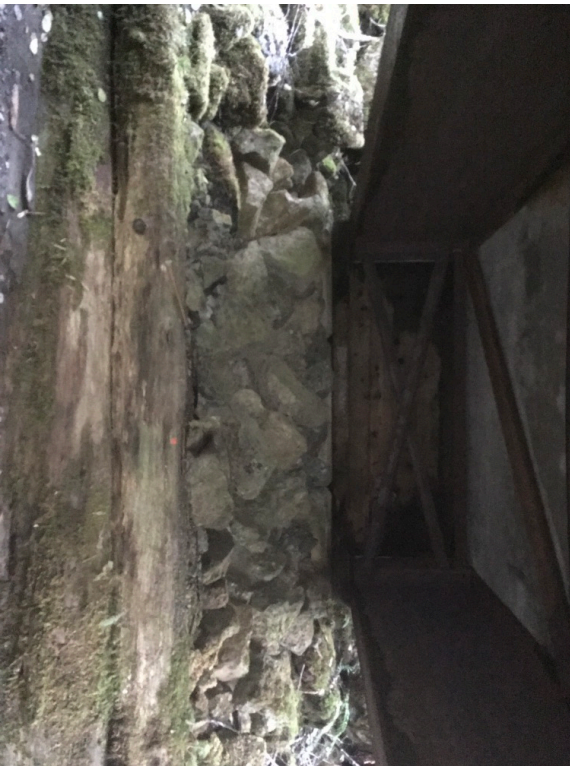
Left Bank Abutment when facing downstream
